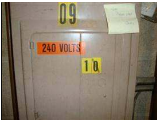
(5) Electrical panel #9 - 240V single phase - OK
