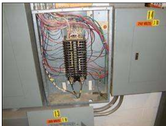
(9) Electrical panel #4 - 240V single phase - double tap wires.
